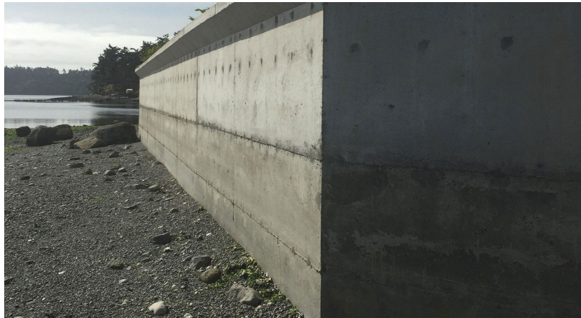
Figure 13. Photo of a bulkhead along Washington’s coast.
