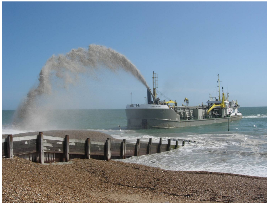
Figure 12. Beach nourishment in progress.
