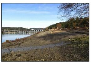
Figure 4. Photo of restored shoreline taken at on March 4, 2013. Bulkhead and fill removed and shoreline topography restored to enhance nearshore habitat for fish and other species.
