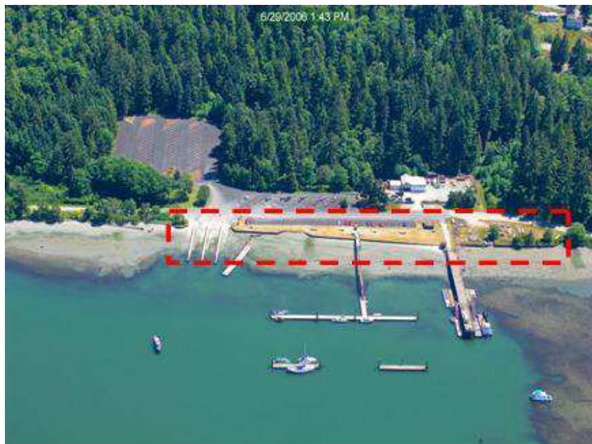
Figure 2. The red box on this 2006 photo outlines the area selected for restoration. It contains four boat launch ramps, a T-shaped public pier used for mooring boats and for fishing, and on the right a Washington State Parks' Marine Crew maintenance pier, closed to the public. The shoreline had been armored with over 600 feet of creosote-contaminated bulkhead which held in place tons of fill imported in the 1970s, covering the upper intertidal beach. The fill created a flat bench planted with grass.
